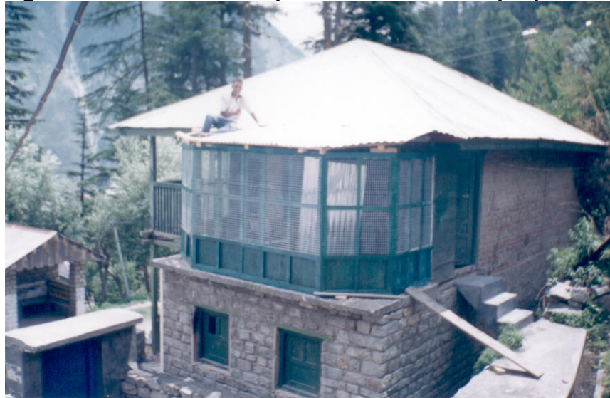
Fig 4 Retrofitting of Women Training Centre in Kinnaur
