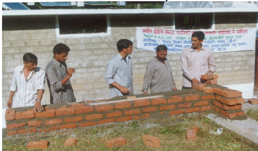
Fig 6. Training of Masons in Cavity wall construction
