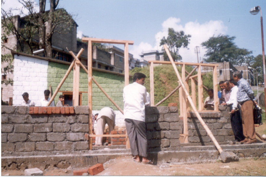
Fig 5. Construction of Passive solar Rural House by Trainee Masons
