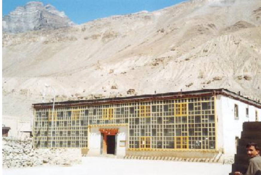
Fig 3 Solar Trombe wall System Tabo monastery, Spiti
