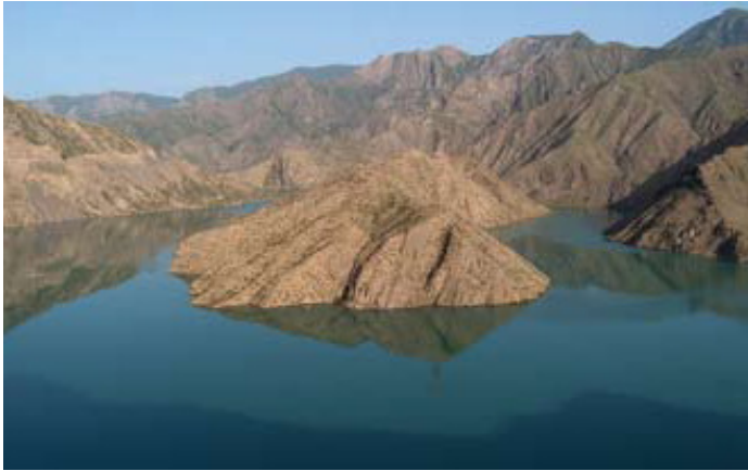
Stored water can be used for energy purposes
